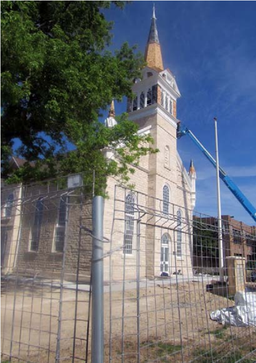
Manti Tabernacle under construction.
