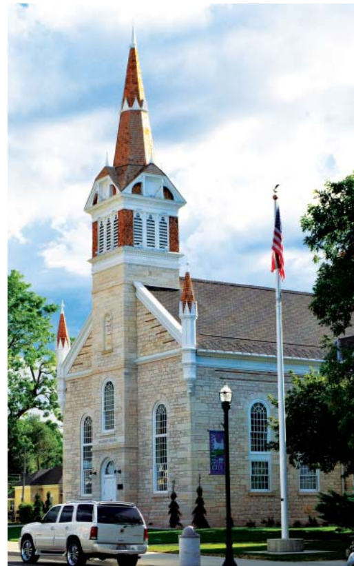
Manti Tabernacle Sept. 2015, after renovations are completed.
