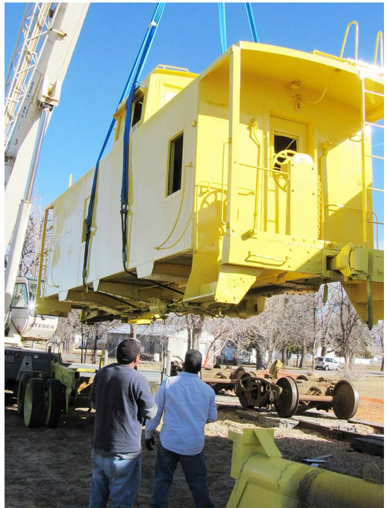
A caboose is hoisted into place at Track 89 North, a railroad resort being constructed on the south end of Mt. Pleasant.
