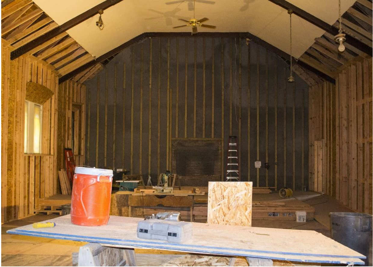
Interior work in progress. (Picture courtesy of Lori Wait)
